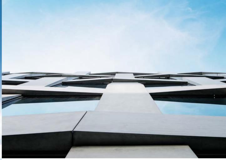
Praga Studios office building Czech Republic | Prague | 2018 investor Praga Studios a.s. | SKANSKA a.s. ADNS Architects acreage GRC 2000 m<sup>2</sup> anchoring Smart – Stud-frame, sprayed anchor invisible surface smooth color light grey 9 ←
